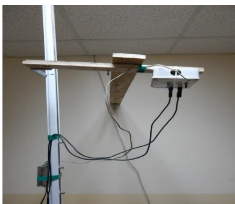
Figure 1. Smoke level measuring device in Volte unite
